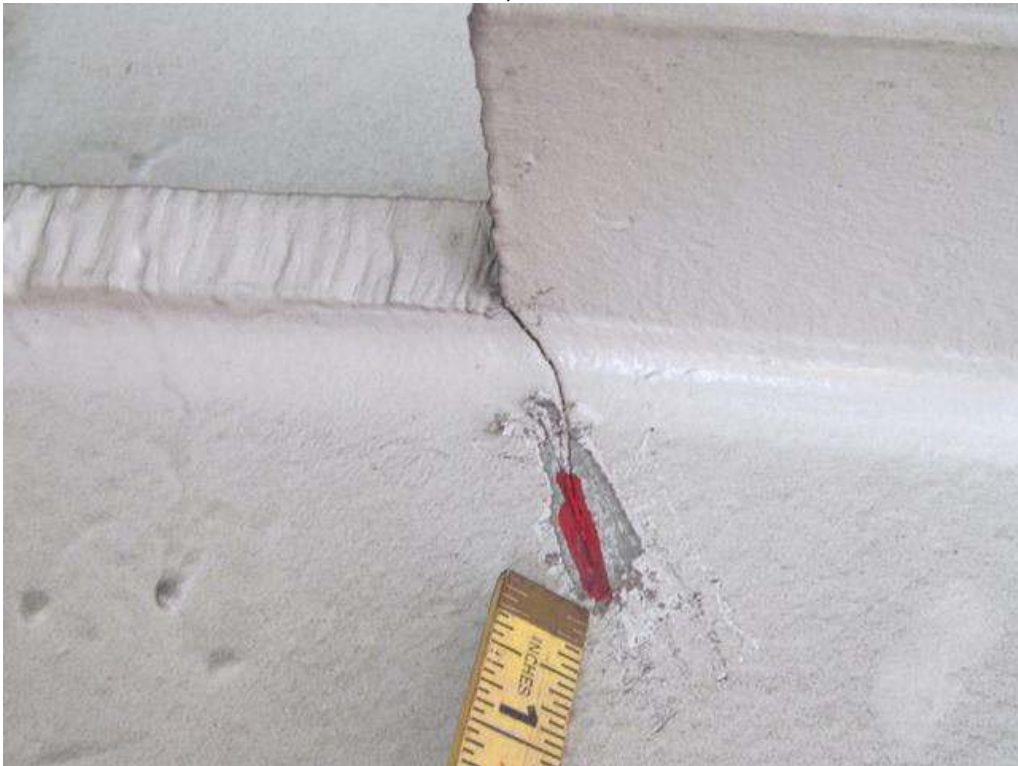
CRACK ( 3" ) IN TOP OF DIAPHRAGM. BEAM 4, SPAN 3
