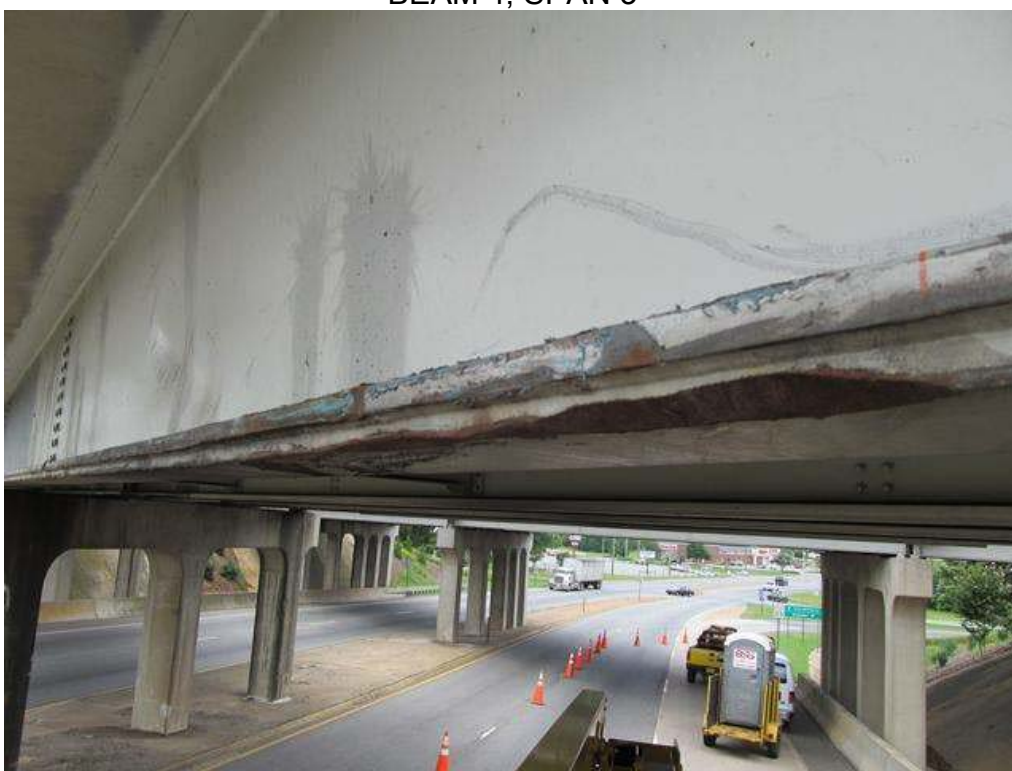
LOOKING AT BEAM 4 FROM BENT 3. BEAM 4 FLANGE AND COVER IS DAMAGED
