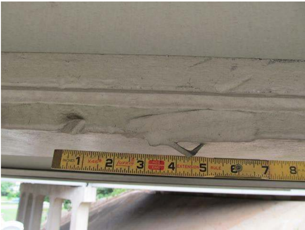
INDENTION ( 1/2" X 1/4" ) IN COVER PLATE @ 35'-1" FROM THE FACE OF BENT 3. BEAM 3, SPAN 3
