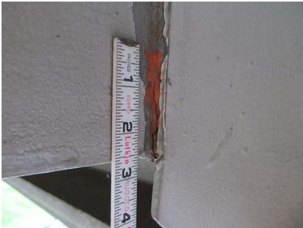
CRACK 2 1/2" LONG IN BOTTOM WELD AT DIAPHRAGM TO BRACKET @ 20'-4" FROM THE FACE OF BENT 3. BEAM 4,
