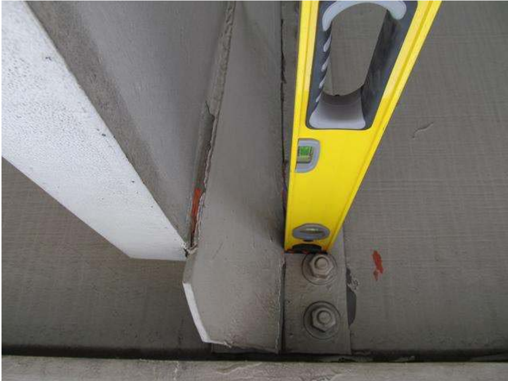
DIAPHRAGM IS BENT 4 1/2" TO THE EAST @ 20'-4" FROM THE FACE OF BENT 3. BEAM 4,
