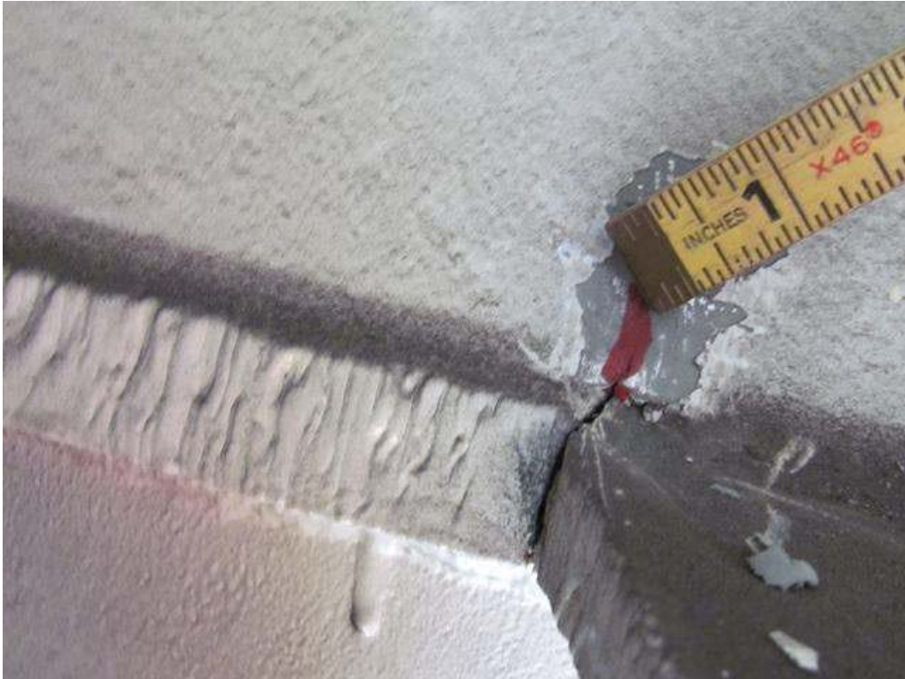
CRACK ( 2" ) IN BOTTOM OF DIAPHRAGM. BEAM 4, SPAN 3
