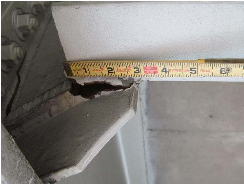
BOTTOM WELD OF DIAPHRAGM HAS A 3" CRACK. BEAM 4, SPAN 3
