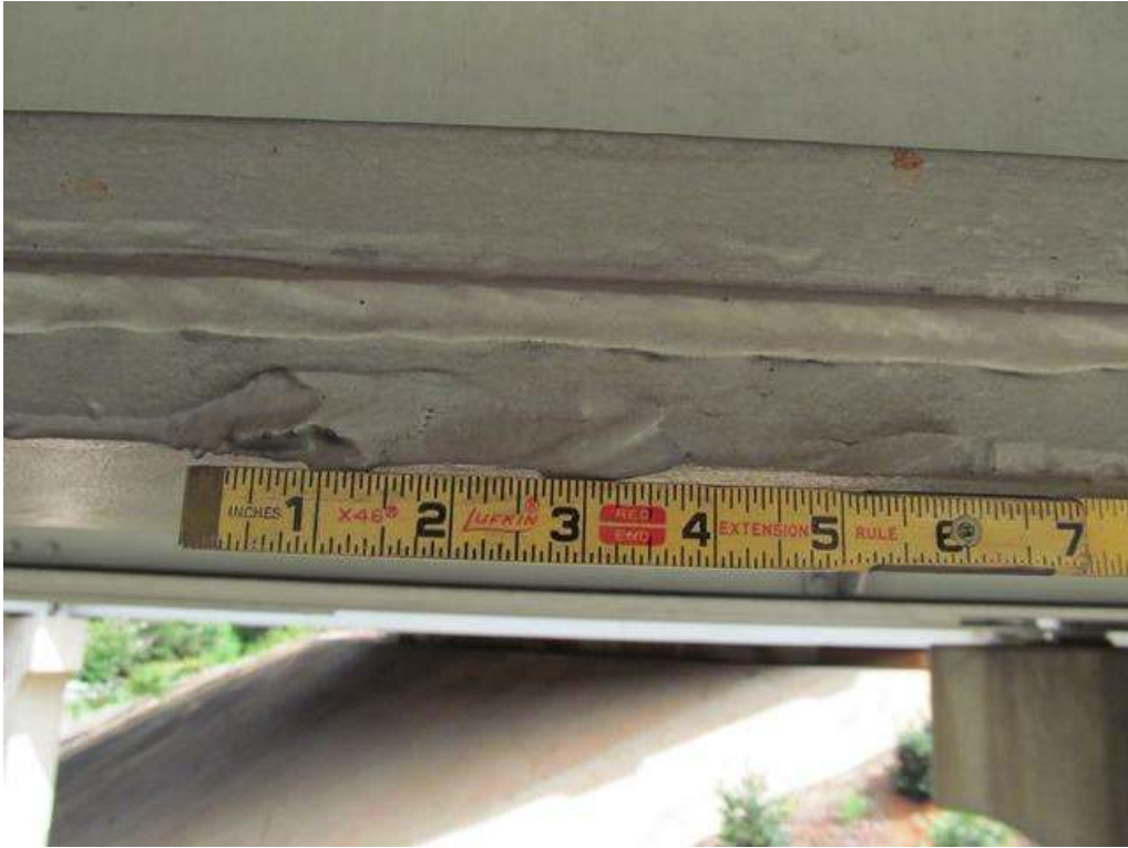
INDENTION ( 6" X 1/4" ) IN COVER PLATE @ 23'-2" FROM THE FACE OF BENT 3. BEAM 3, SPAN 3
