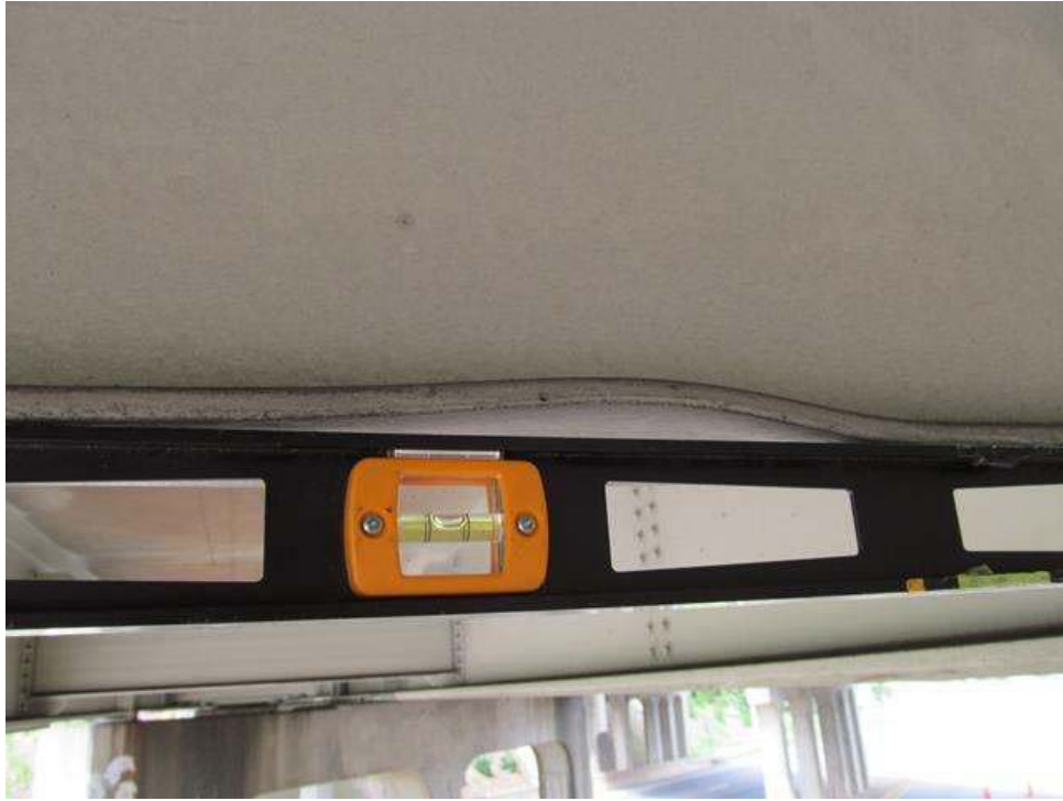
DIAPHRAGM IS BENT ( \frac{3}{4} " ) UPWARD AT 4'-0" FROM BEAM 4 @ 37'-4" FROM THE FACE OF BENT 3. BEAM 4, SPAN 3
