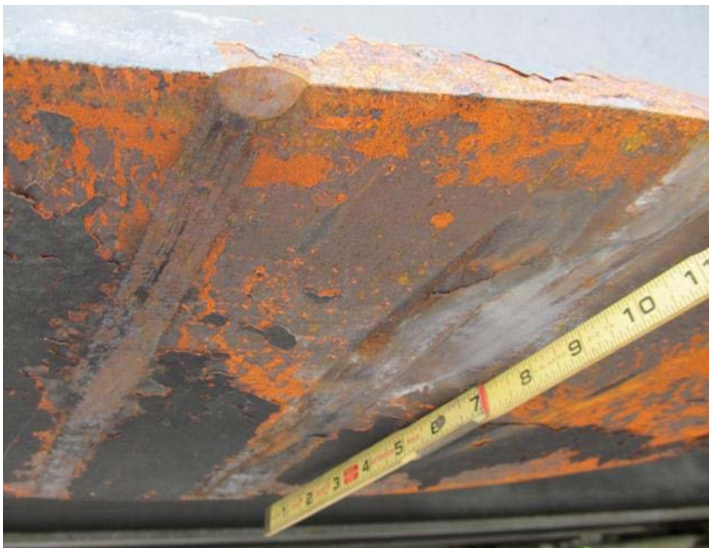
GOUGE IN BEAM 6 AT 14'-1"
