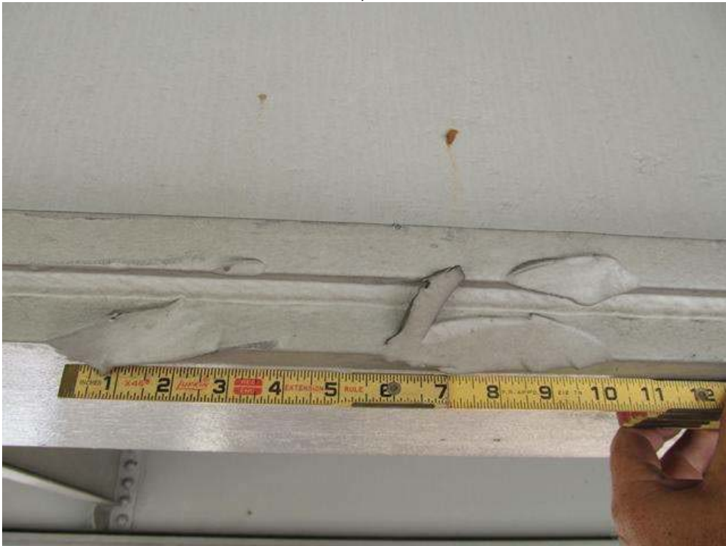
POINT OF IMPACT ON BEAM 2 IS 34'-2" FROM THE FACE OF BENT 3. BEAM 2, SPAN 3
