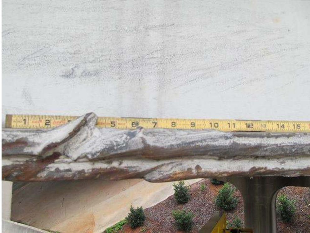
POINT OF IMPACT ON BEAM 4 IS 33'-10" FROM THE FACE OF BENT 3.
