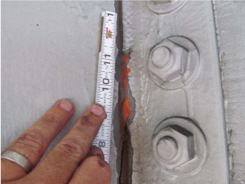
CRACK 11" LONG AT THE BOTTOM OF DIAPHRAGM BRACKET @ 20'-4" FROM THE FACE OF BENT 3. BEAM 4,
