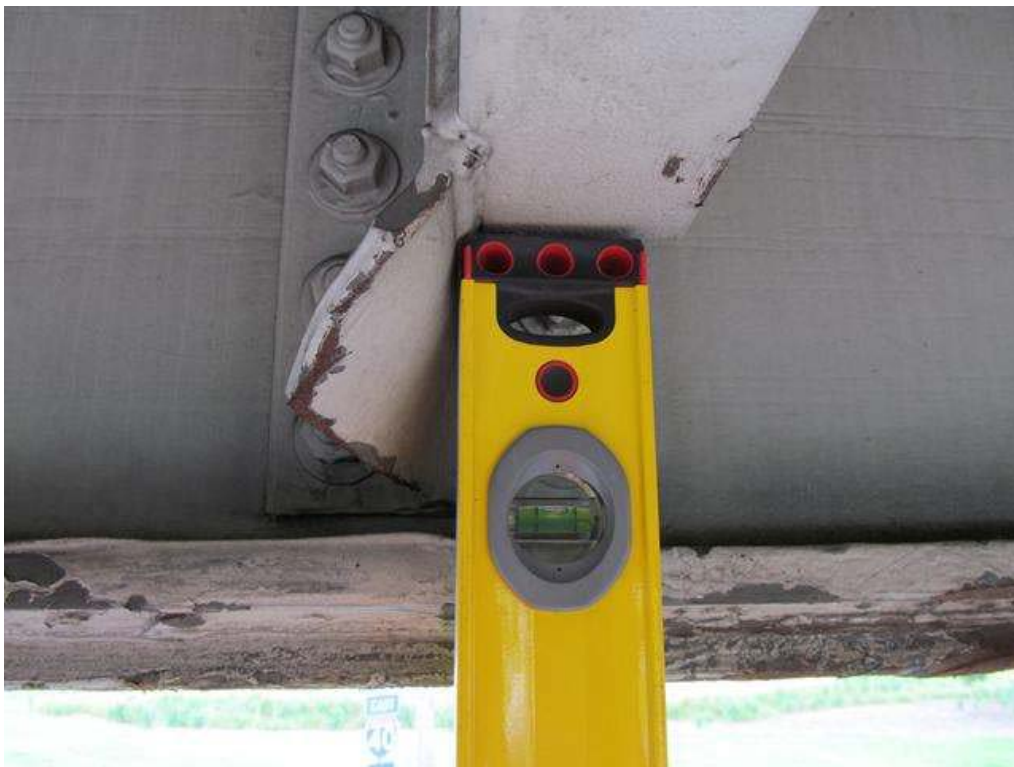
TOP AND BOTTOM OF DIAPHRAGM BRACKET IS BENT UP TO 2" TO THE EAST. OUT OF PLUMB @ 18'-2" FROM THE FACE OF BENT 2. BEAM 4, SPAN 2
