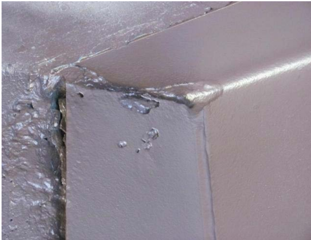
STIFFNER ON GIRDER #8 NO WELD CONDITIONS FOUND.
