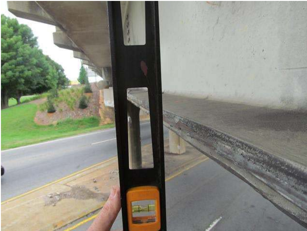
BEAM 4 IS OUT OF PLUMB ( 1 \frac{7}{8} ") TO THE NORTH @ 30'-0" FROM THE FACE OF BENT 3. BEAM 4,
