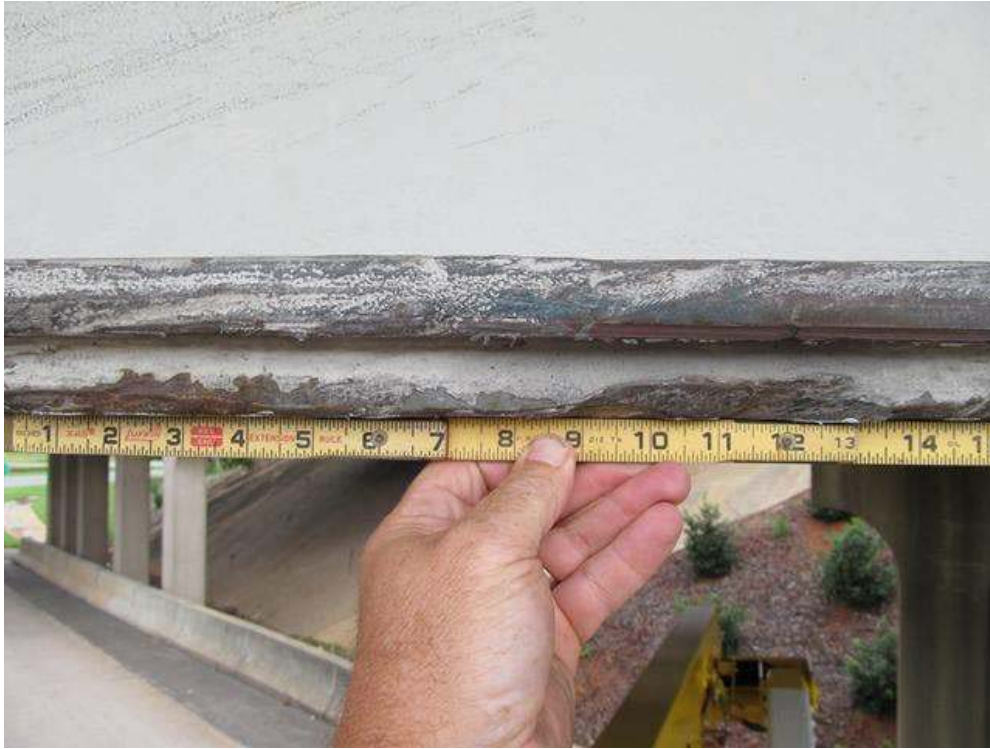
INDENTION ( 16" X 1/2" ) IN COVER PLATE @ 32'-0" FROM THE FACE OF BENT 3. BEAM 4,
